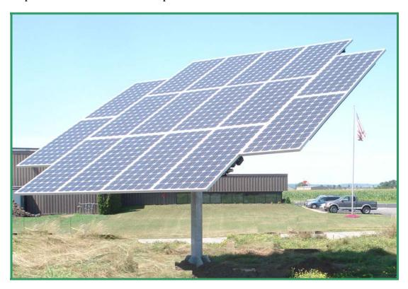
Our fixed racking system has an optional manual adjustment available. This adjustment will tilt your solar panels so they can maximize the sun's rays whether it is the longest day of the year, or the shortest day.
