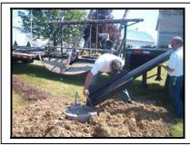
**2.3** Once the post is sitting on the concrete pad, fasten and tighten the nuts to the J-bolts.
