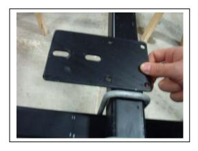
The picture on the left is the panel plate and also shows a white line which represents where the panels will meet on the plate. The white line is centered on the 2x6. The oval holes are used to secure the panels.
