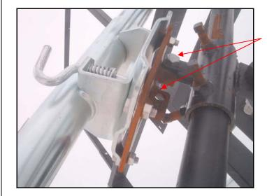
Fasten plate to Elevation tube
